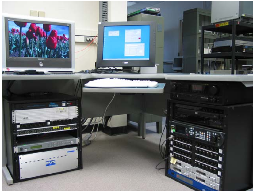
Uncompressed HDTV Equipment
