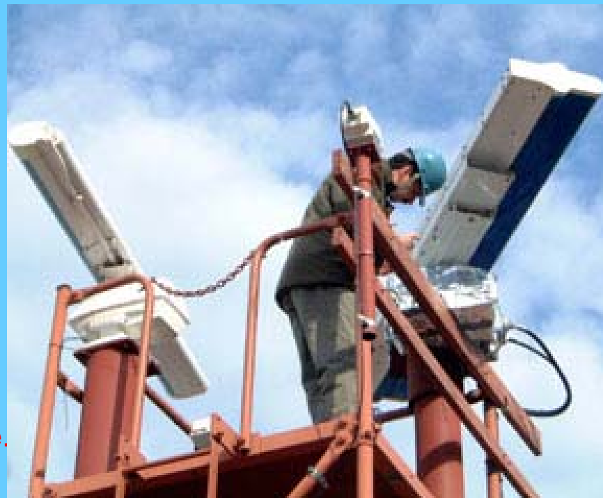
OSM engineer preparing a maritime radar for signal injection at Curtis Bay Coast Guard Station near Baltimore.
