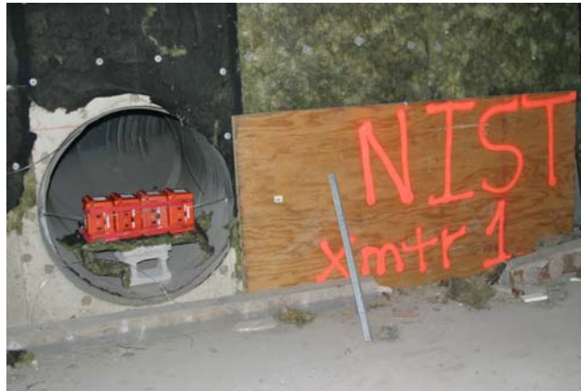
Ventilation duct Washington, DC
