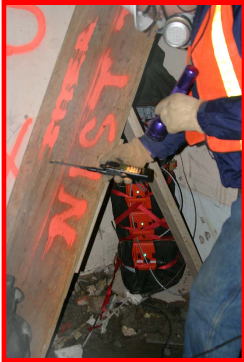
Transmitters are secured to the wall and protected from falling debris by a board
