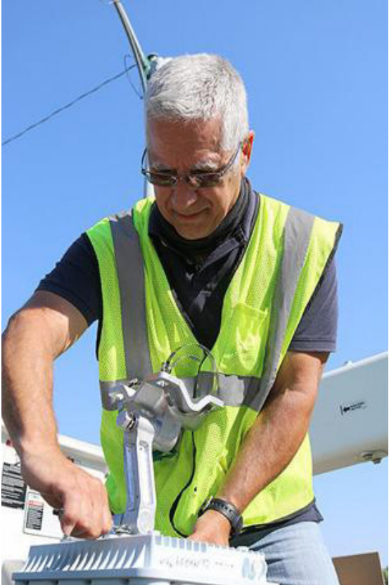
A bracket being mounted on a SmartWave AP. Source: Council Bluffs School District
