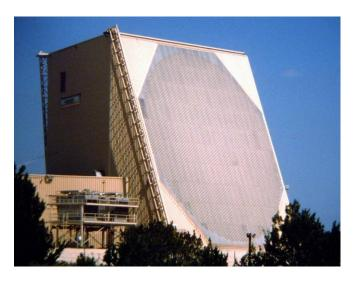
Figure 39. FPS-123(V) PAVE PAWS missile and space surveillance radar system (courtesy: USAF).
