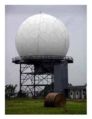
Figure 42. Long-range ARSR (antenna is encapsulated by radome).
