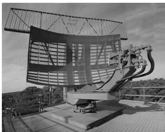
Figure 5-7. Air Traffic Control Radar Beacon Antenna
