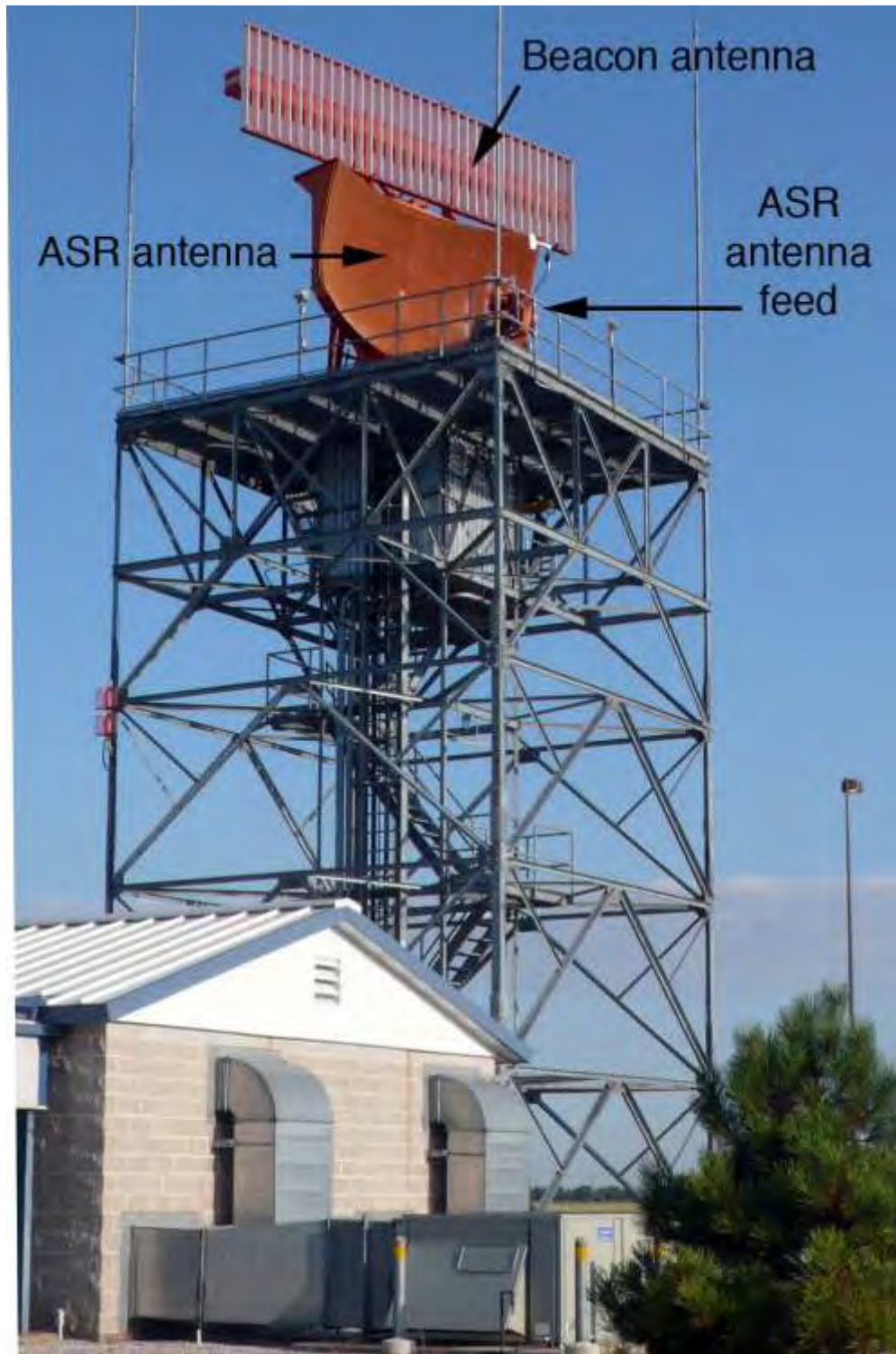
Figure C-1. An airport surveillance radar antenna (here an ASR-11) as typically deployed on a tower. The beacon antenna is part of an electronically separate system.
