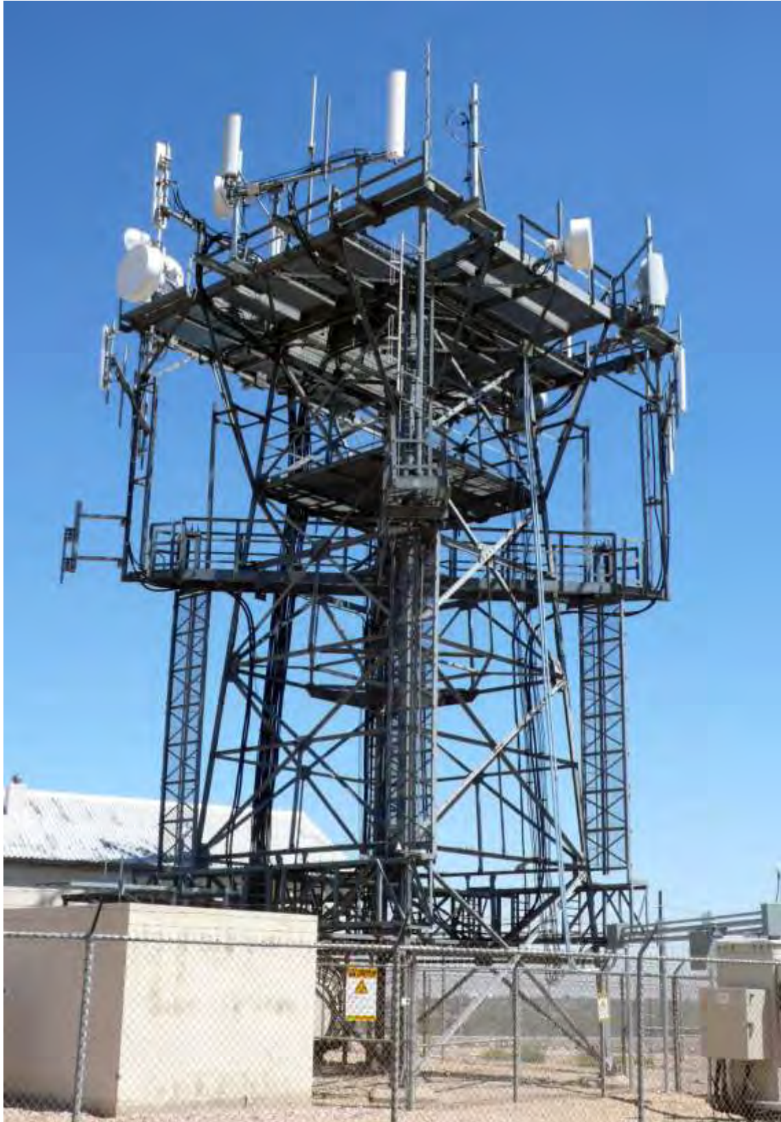
Figure 15. An example of a tower on which are mounted antennas for a variety of communication systems, including BRS, at Broomfield, Colorado. Photo by author Sanders.
