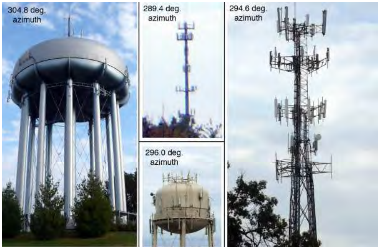
Figure 53. Images of four Grand Rapids BRS/EBS towers where the signals shown in Figures 41–44 were transmitted. Azimuths are as measured from the Grand Rapids NEXRAD station location. Photos by author Sanders.
