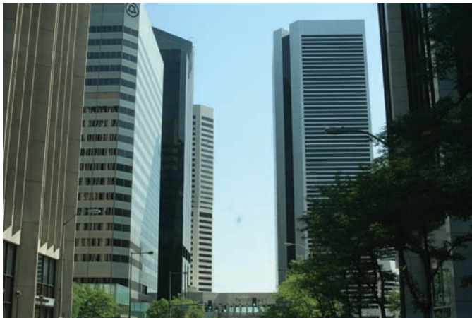
Figure 1. An “urban canyon” contains a large variety of materials, angles and shapes that can reflect or scatter radio waves and present one type of challenge for propagation modeling.
