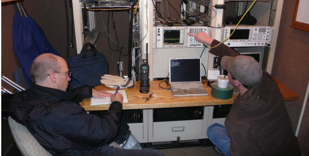
Figure 2. ITS engineers Frank Sanders (left) and Geoffrey Sanders (no relation) perform field tests to verify that 5 GHz U-NII devices with newly-developed firmware correctly detect TDWR signals. Photo by John E. Carroll.
