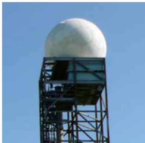
FPS-124 radar on which ITS performed emission measurements. Photo by Frank Sanders.
