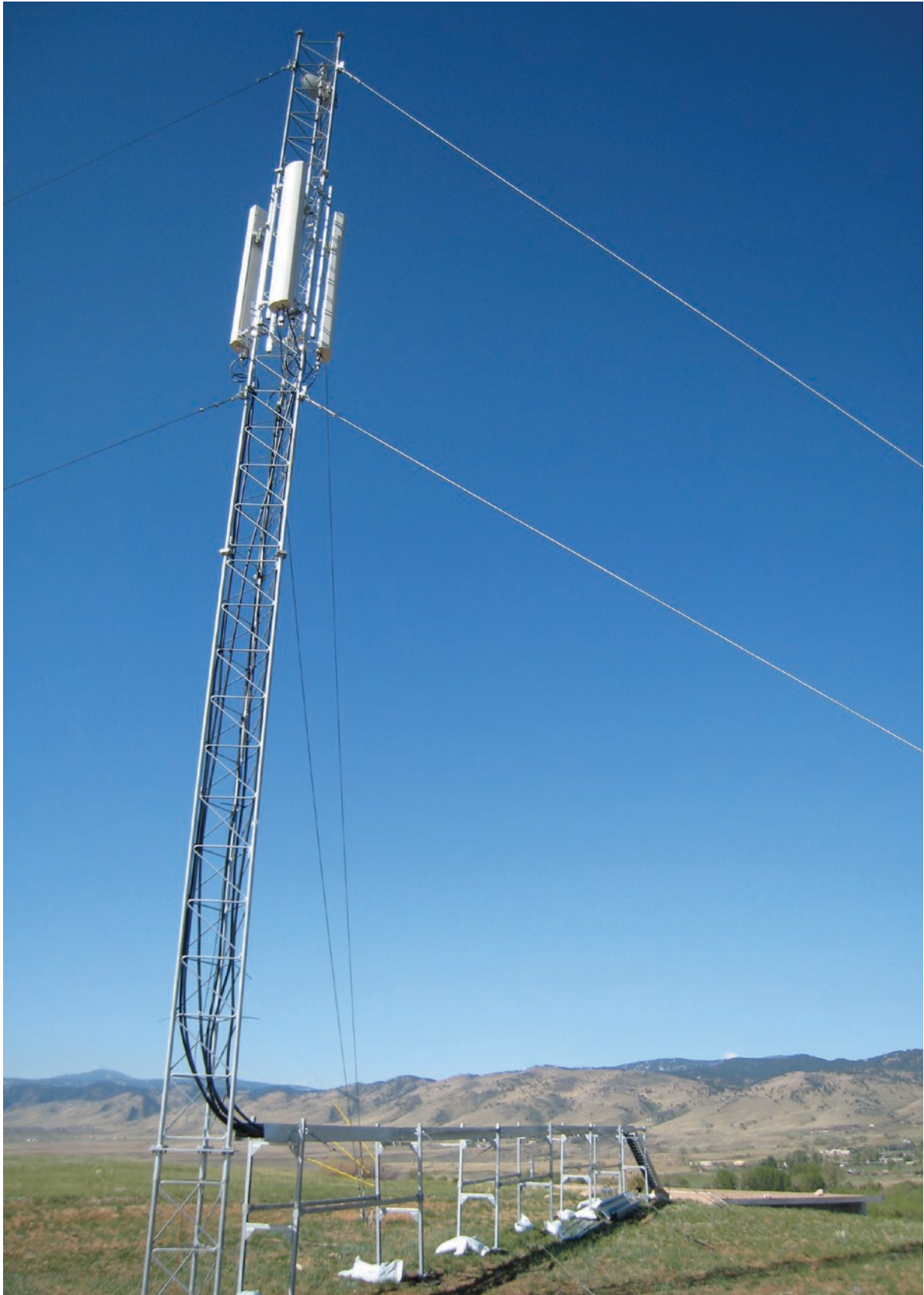
One of the two fixed LTE transmitters used for over-the-air testing in the Public Safety 700 MHz Broadband Demonstration Network. This one is located at the Table Mountain Field Site and Radio Quiet Zone. Photo by Ken Tilley.
