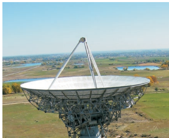
One of the two 18.3 meter (60 foot) parabolic dish antennas at the Table Mountain Field Site..
