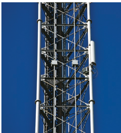
A PSCR Broadband Demonstration Network antenna panel (right) mounted at 84 meters on this 300 meter tower, plays a role in RF interface bandwidth testing. Photo by Ken Tilley.
