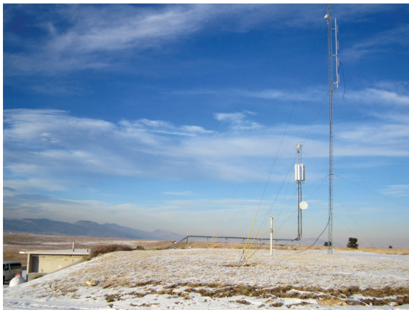
Antenna towers at the Table Mountain Field Site support one of three fixed nodes on the Public Safety Broadband Demonstration Network. The white cylinders on the tower on the left are an array of 700 MHz LTE antennas; below that a microwave antenna connects one field site to the other. Other antennas support different communication systems for OTA testing. Photo by Jaydee Griffith.
