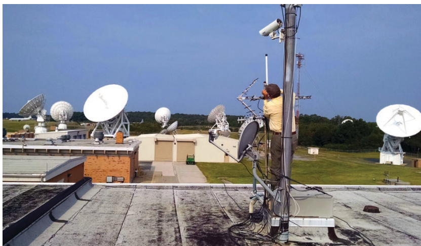
ITS engineer Frank Sanders installs a monitoring antenna at the NOAA/NESDIS CDAS. Photo by David Franc.
