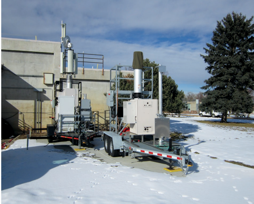
Two cell-on-wheels (COW) units can extend the reach of the fixed nodes on the Public Safety Broadband Demonstration Network. Photo by Jaydee Griffith.
