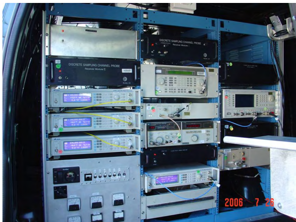
Figure 5. Interior view of the receiver mounted in the van.
