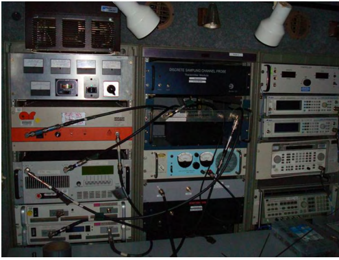
Fig. 2. Interior view of the transmitter equipment rack.
