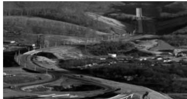
Figure 9 Aerial view of the Smart Road - Blacksburg, VA
