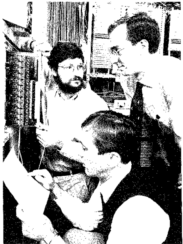
Tim Butler, Darren Smith, and Rob Debolt Check ITS LAN Connections
