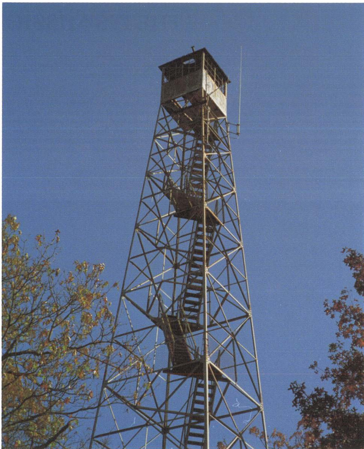
Forest Service Fire Lookout Tower with Land Mobile Radio Antenna Mounted Near the Cab. See Advanced Systems Planning, Page 42. Photograph by W.R. Rust.
