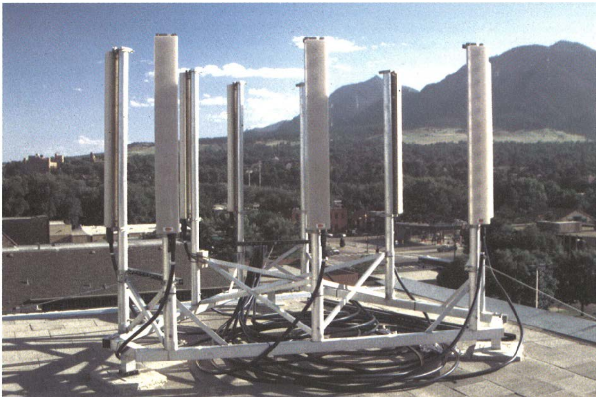
Antenna of a PCS base station in the Boulder Industry Test Bed (photograph by F. Sanders).
