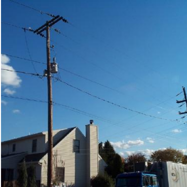
Figure 2-44: Transition from 3-phase to 2-phase conductors
