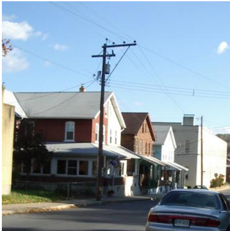
Figure 2-41: Offset 3-phase power line conductors
