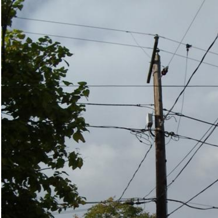
Figure 2-42: Offset 2-phase power line conductors
