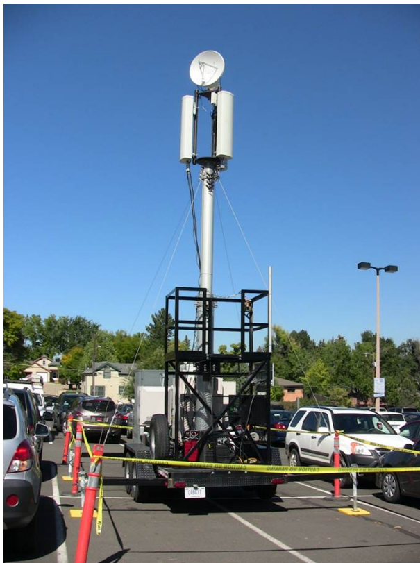
Figure 30. COW placement in the parking lot. Note the microwave backhaul dish antenna on the top of the mast.
