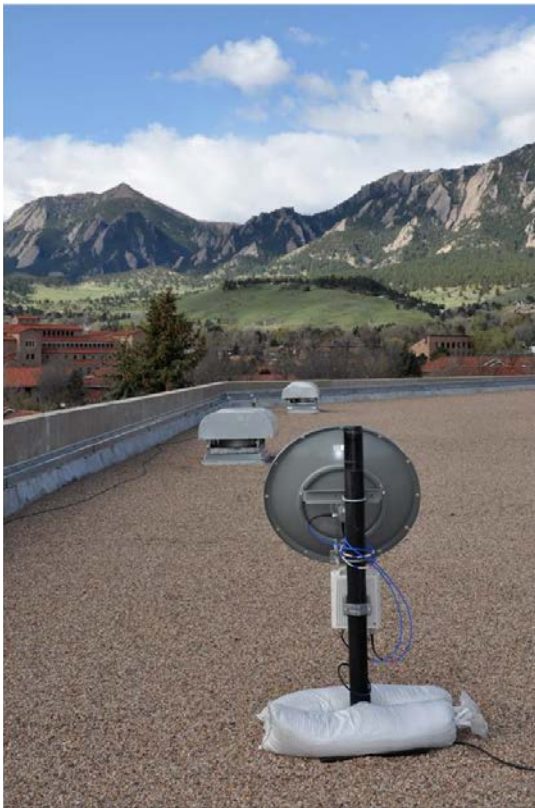
Figure 180. Microwave backhaul antenna and transceiver bore sighted at the Green Mountain station.
