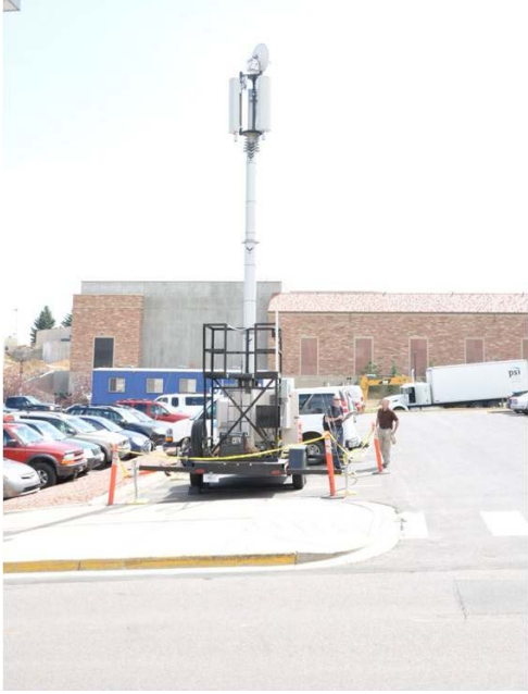
Figure 174. The COW deployment viewed from the north. The COW antenna is bore sighted directly at the north wall of the CEC.
