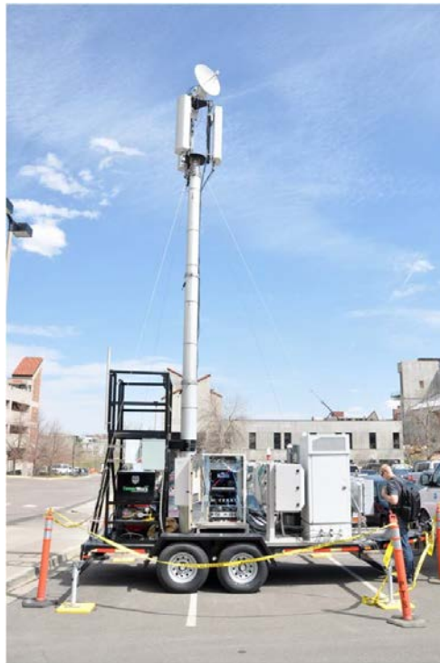
Figure 175. The COW deployment viewed from the west. The dish antenna is the microwave backhaul and it is aimed directly at the Green Mountain eNB, where the companion link system is located.
