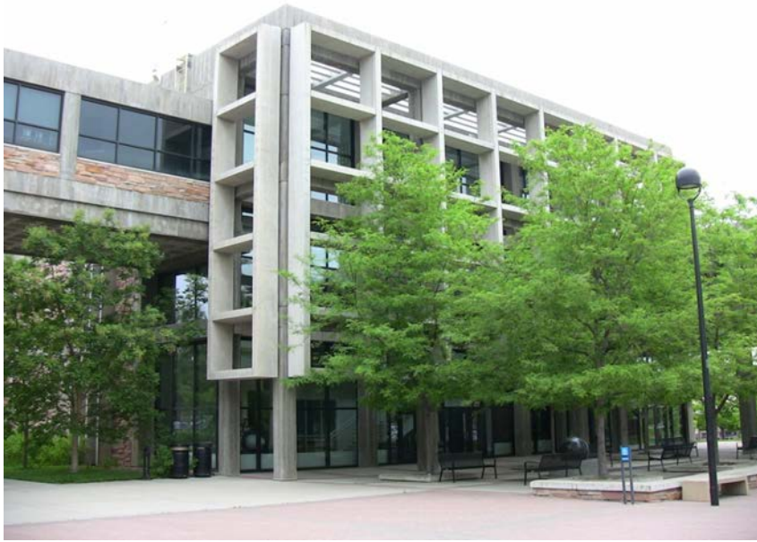
Figure 4. The main entrance to the Discovery Learning Center. Note the open concrete framework backed by a glass wall.
