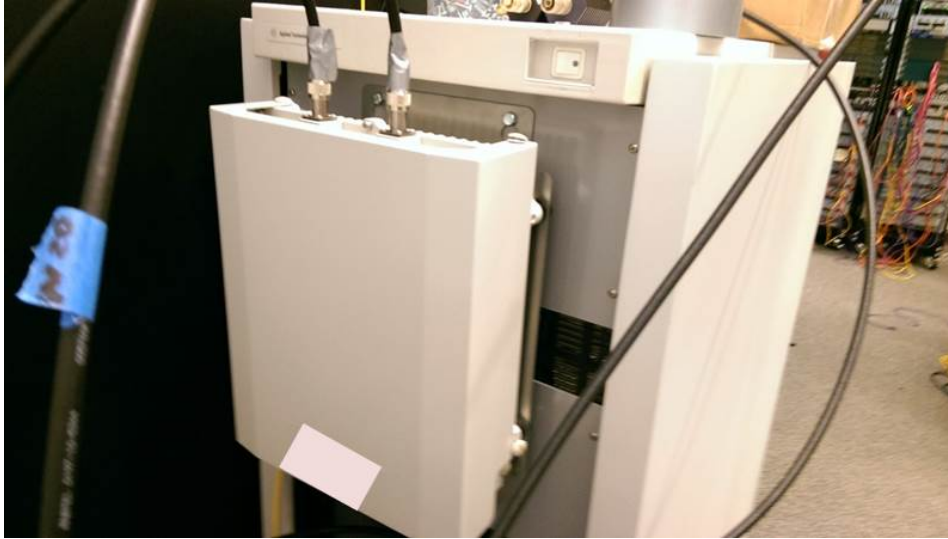
Figure 27. Small cell feeding the DAS network (SCDAS).
