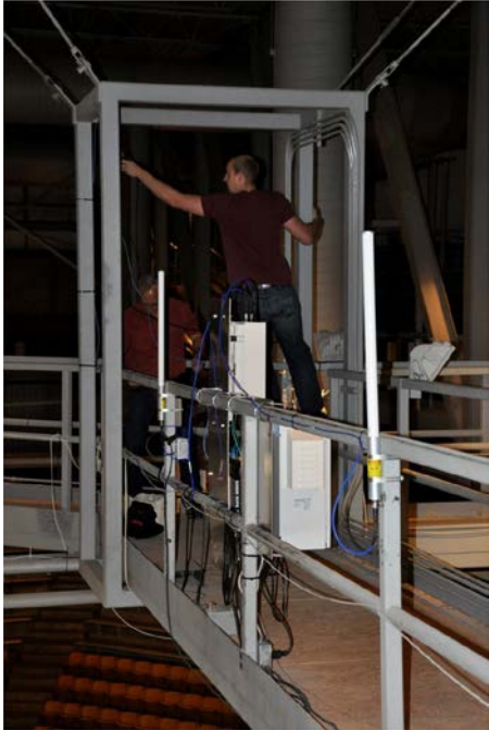
Figure 179. A PSCR engineer installs power over Ethernet cable from the microwave backhaul to the router.
