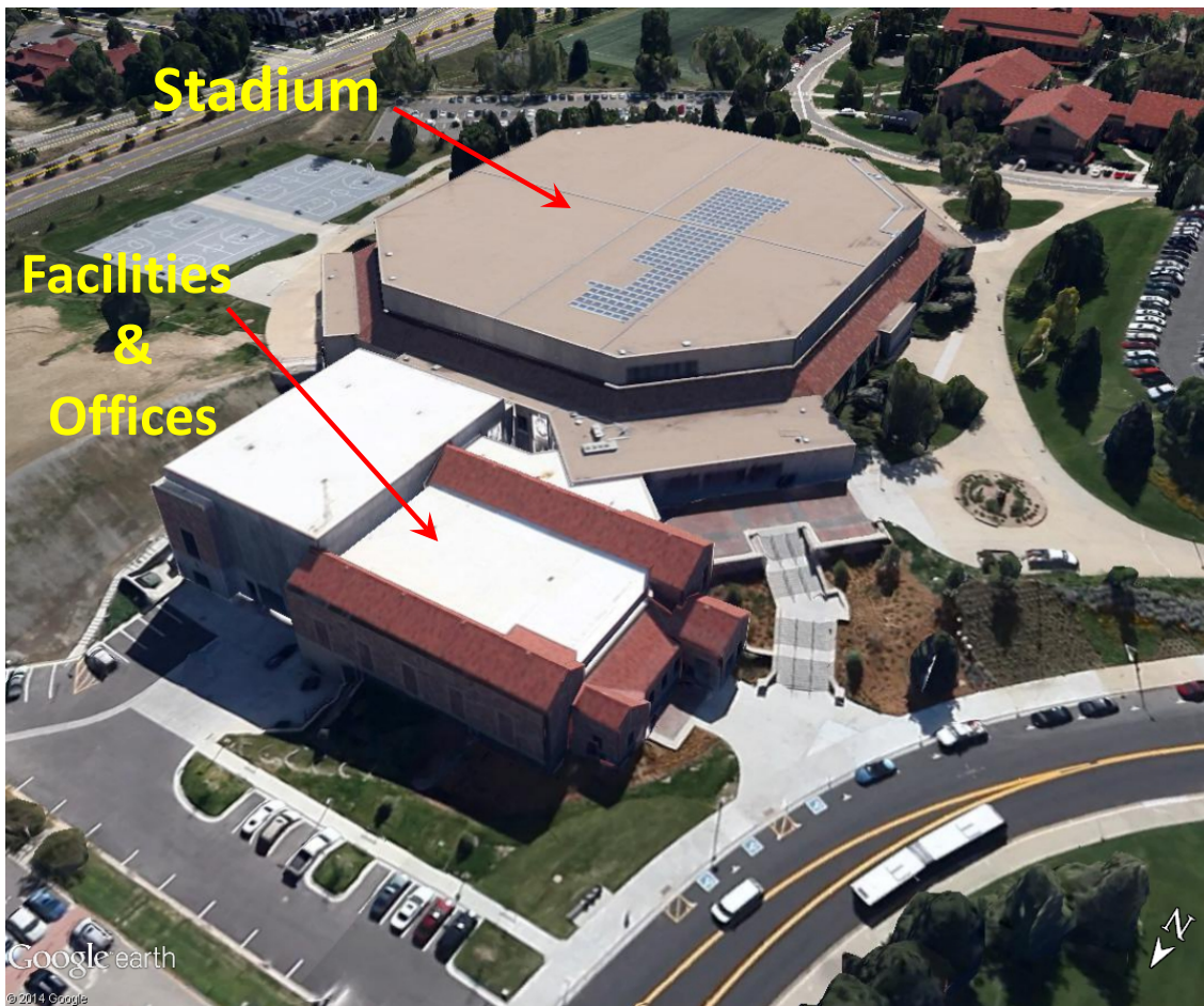
Figure 164. Aerial view of the Coors Event Center showing both the stadium and facilities/offices sections (FOS).
