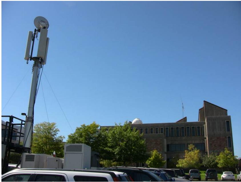
Figure 29. COW deployment in a parking lot located directly east of the DLC.
