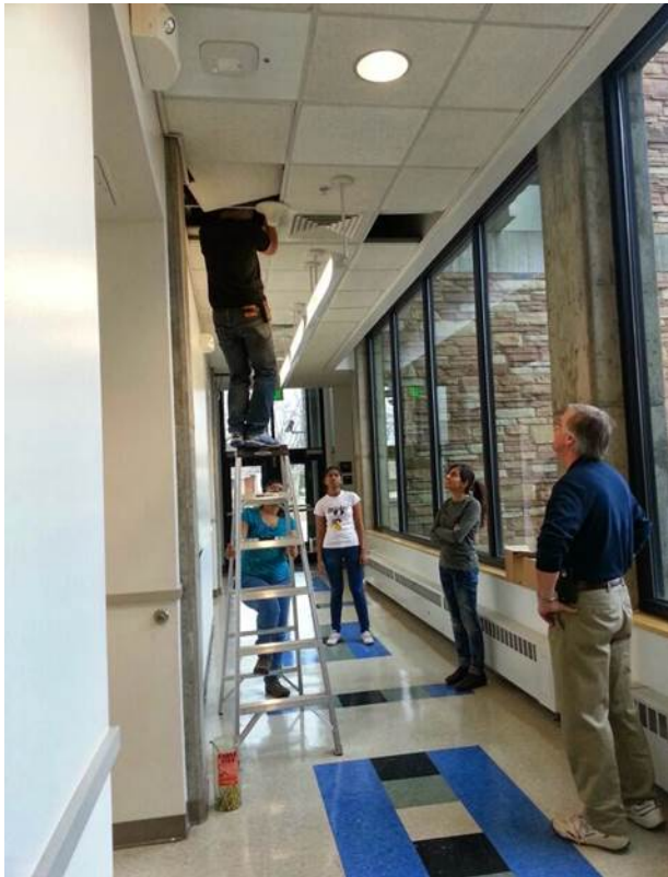
Figure 26. Installation of the DAS system at the DLC.
