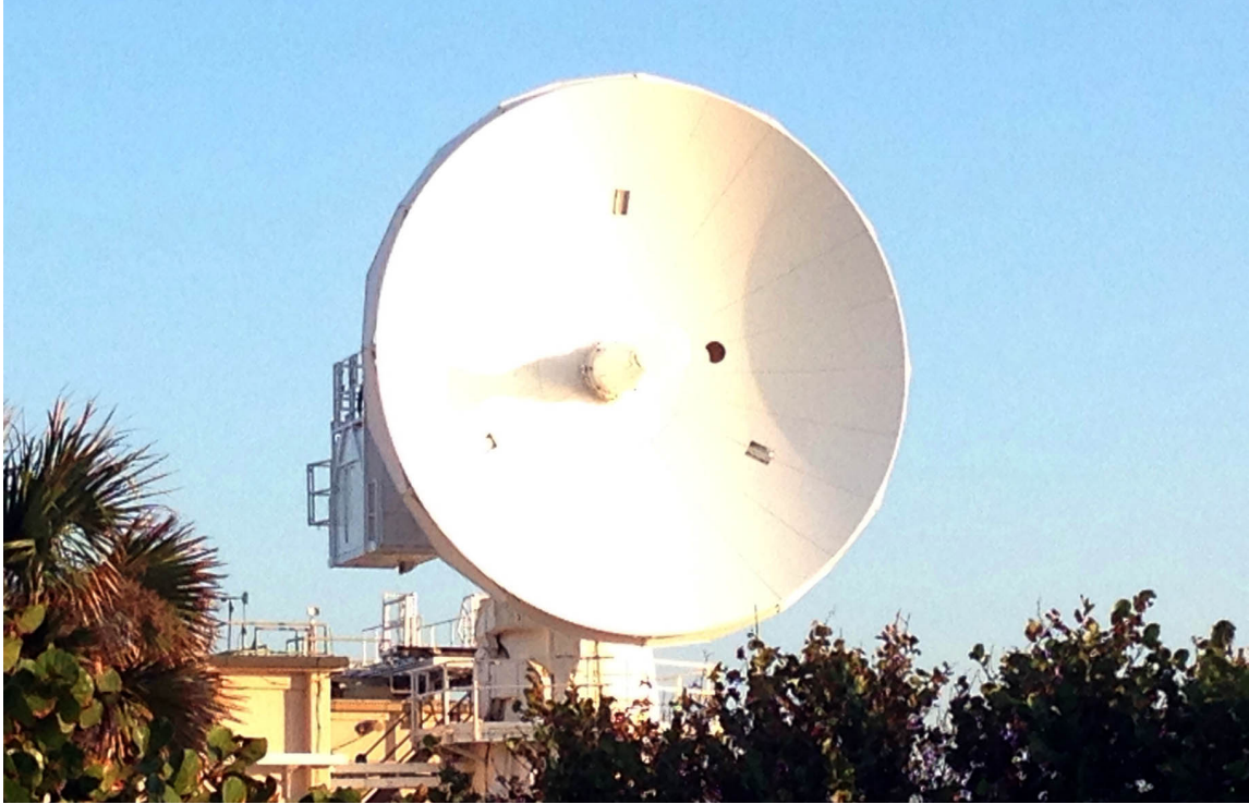
Figure 5. A RIR antenna (8.8 m diameter). Note three strut support points for an earlier-generation RF feed. Circular aperture at right is for a co-axial telescopic camera.
