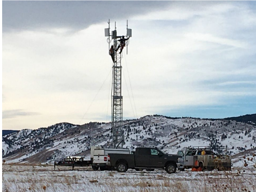
Figure 34. One of the pair of Radio 1 CoWs at Table Mountain, with a set of three lower C-band (3300–3600 MHz) MIMO panels at the “normal” 12 m (40 ft) height.
