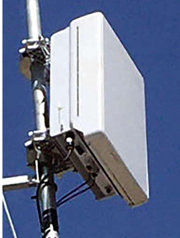
Figure 18. A MIMO 64T64R transmitter-receiver box for a US n77 band 5G base station. It is an integrated, weather-sealed unit with connectors on the lower edge for power and data.
