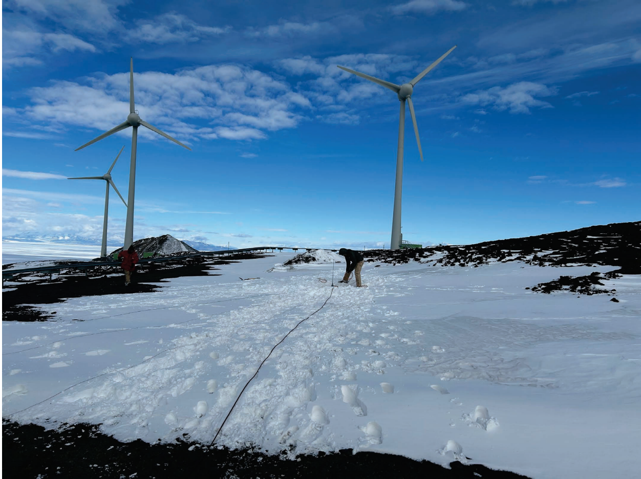
Figure 60. Setting up radial ground plane at MTRS-2 with three wind generators in background. (Credit: Robert Achatz)
