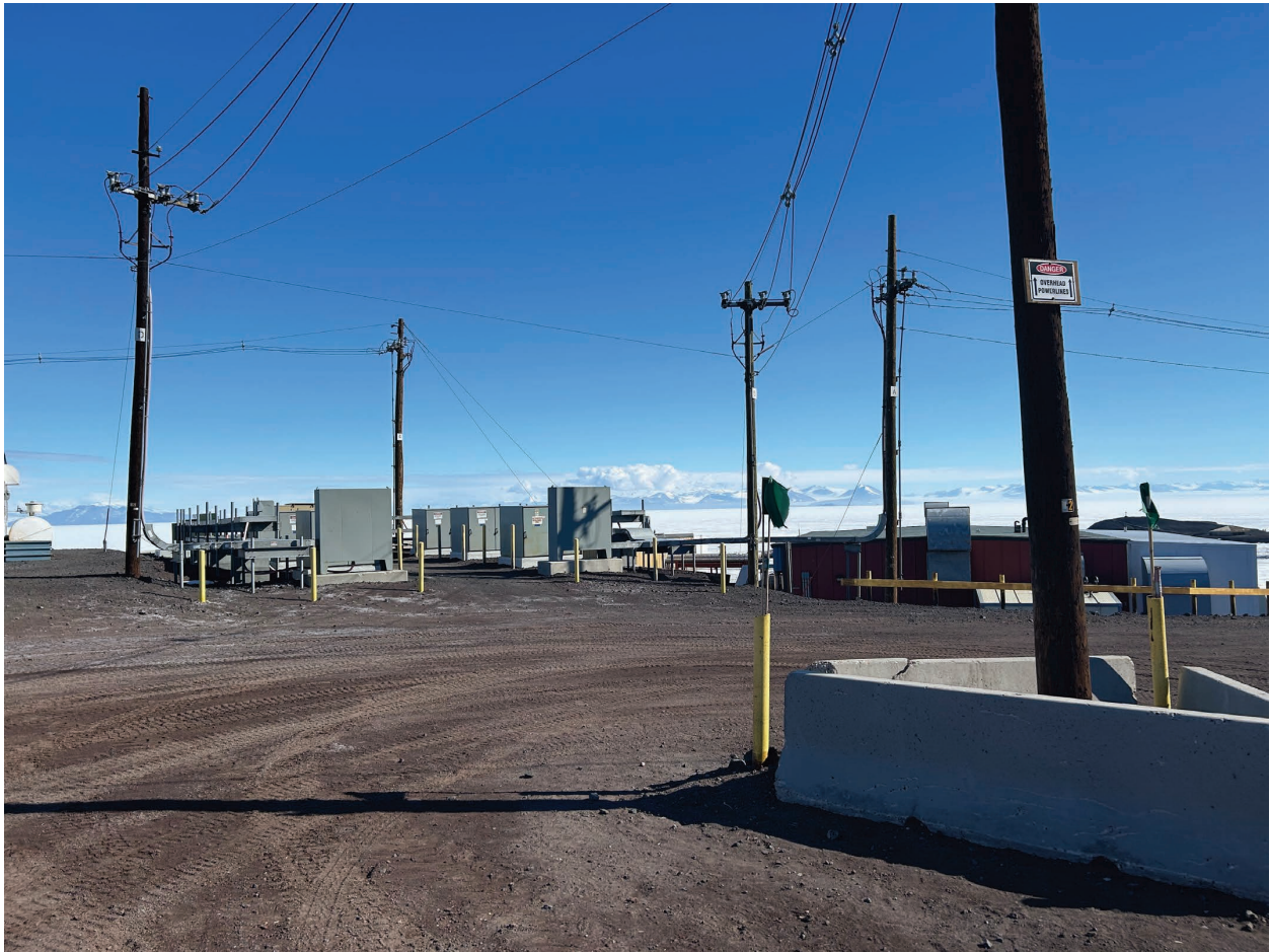
Figure 3. Power lines and power distribution equipment in gray metal cabinets in front of MS power generator buildings 196 and 198. (Credit: Robert Achatz)
