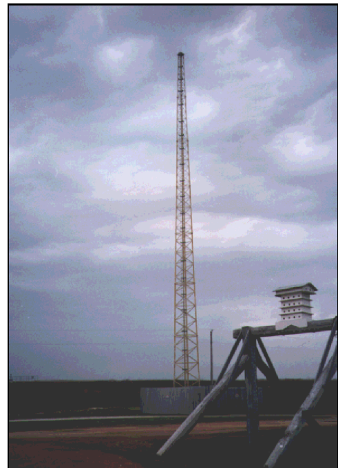
Figure 4. Transmitter at Mobile Point, Alabama.
