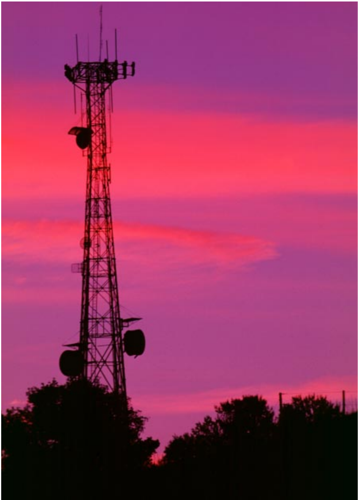
A cellular telephone antenna near Boulder, Colorado (photograph by D.J. Atkinson).
