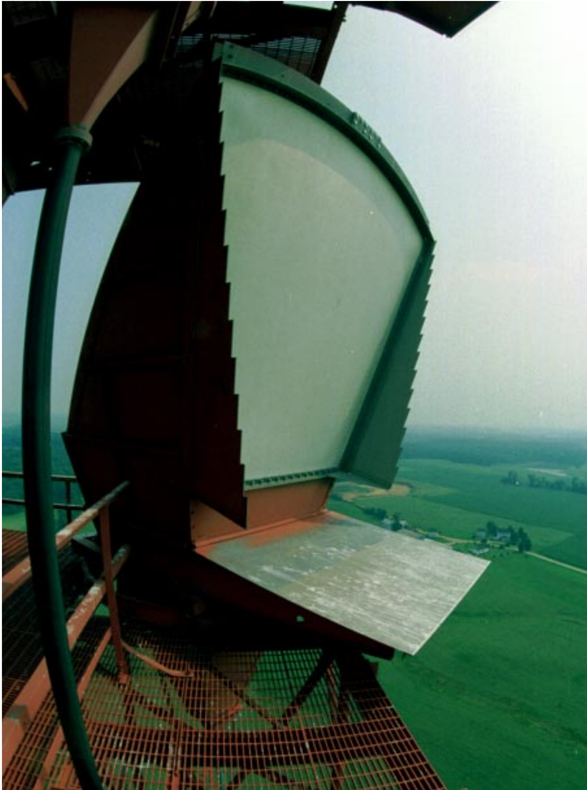
This point-to-point microwave link has been vacated; the spectrum it used to occupy may become available for new technologies and services. The Institute provides spectrum engineering support to Government and industry in rapidly evolving telecommunications fields (photograph by F.H. Sanders).
