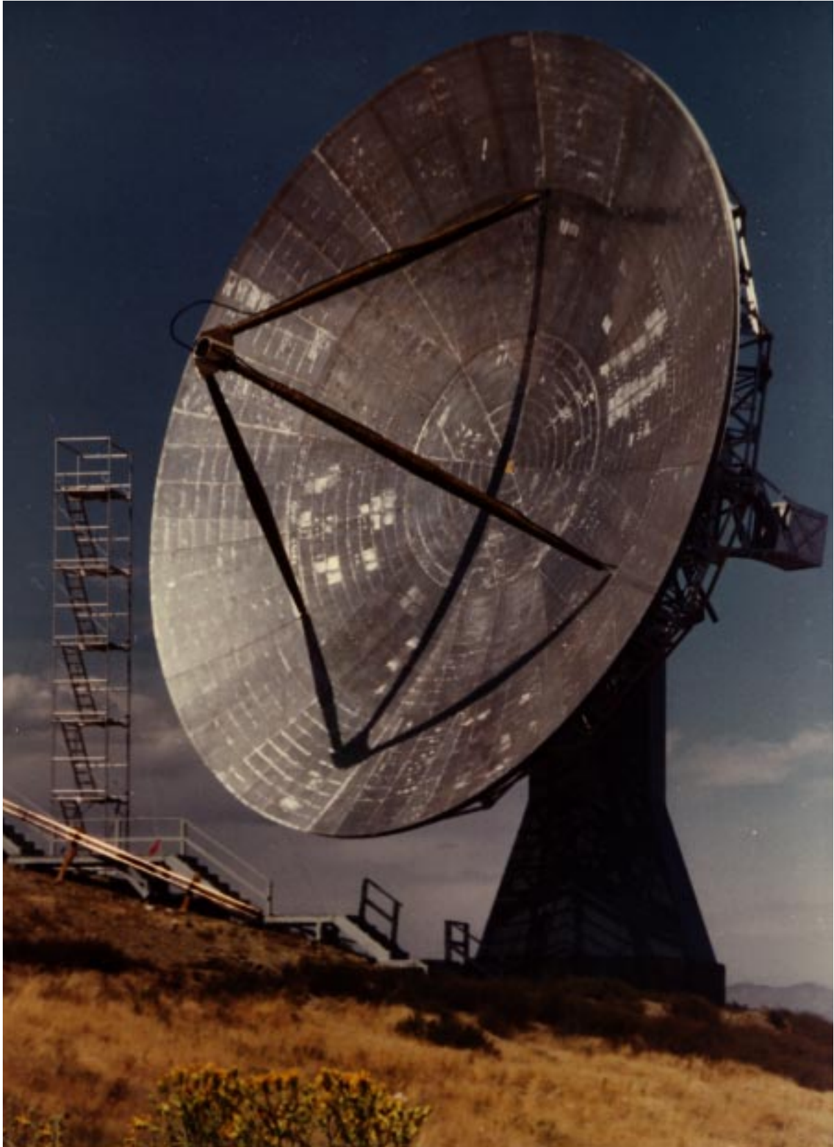
Sixty-ft antenna at the ITS Table Mountain Radio Test Facility.
