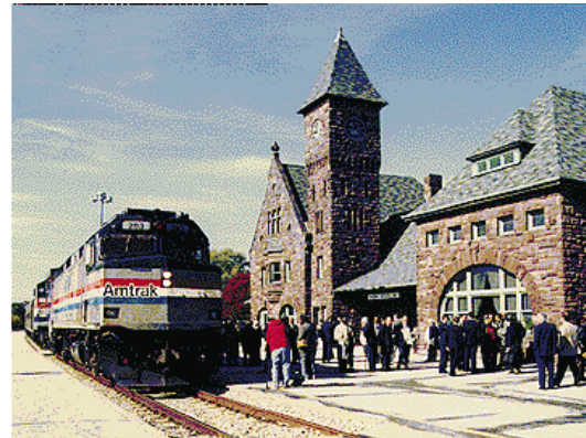
Amtrak station at Niles, Michigan (image courtesy of G.E. Transportation Systems).
