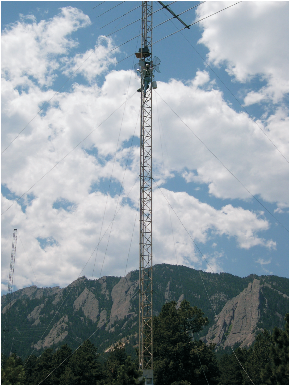
Telecommunications Engineering, Analysis, and Modeling Division engineer installing an antenna at the Green Mountain Mesa field site, part of the short & long range wireless test links (photograph by C. Redding).
