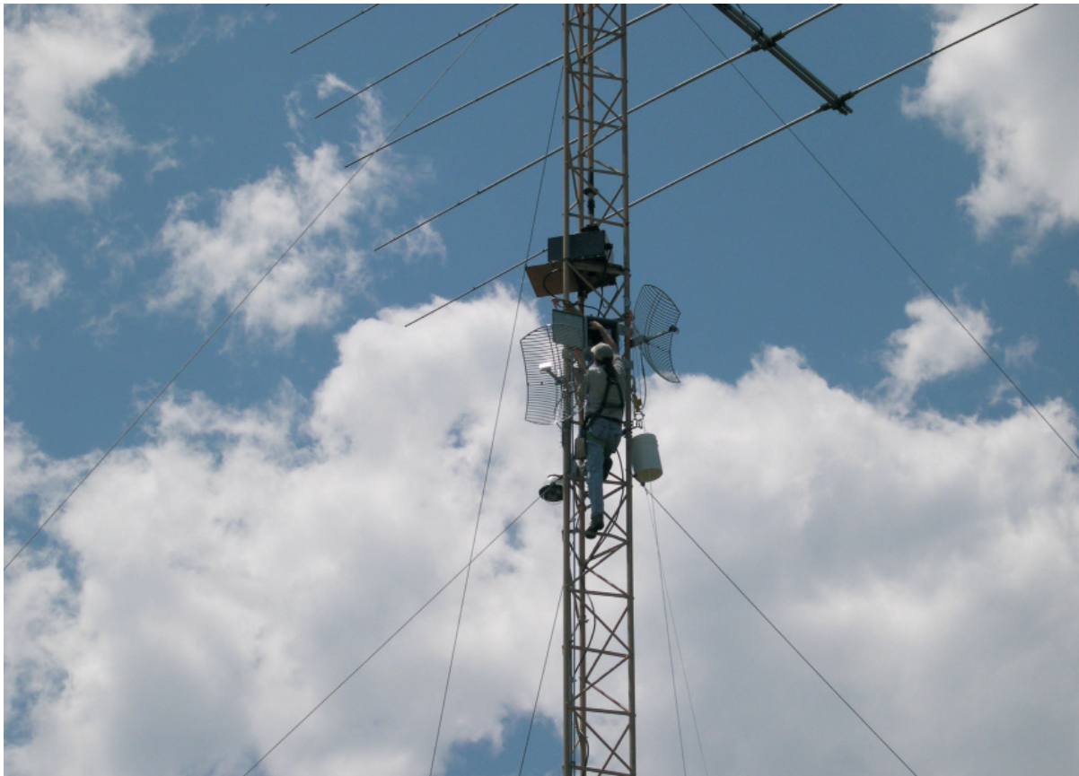
ITS engineer installing an antenna at the Green Mountain Mesa field site (photograph by C. Redding).
