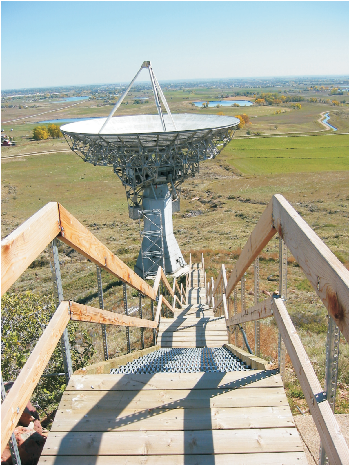
Newly installed stairs leading to an 18.3-meter (60-foot) parabolic dish antenna at the Table Mountain field site (photograph by J.D. Ewan).
