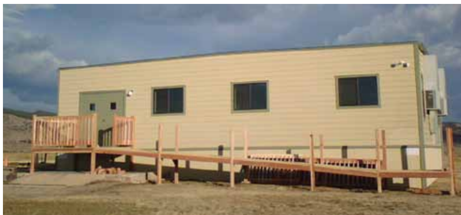
Many facilities at Table Mountain, like this research station, are being upgraded as a part of a modernization project at the site (photograph by J.W. Allen).
