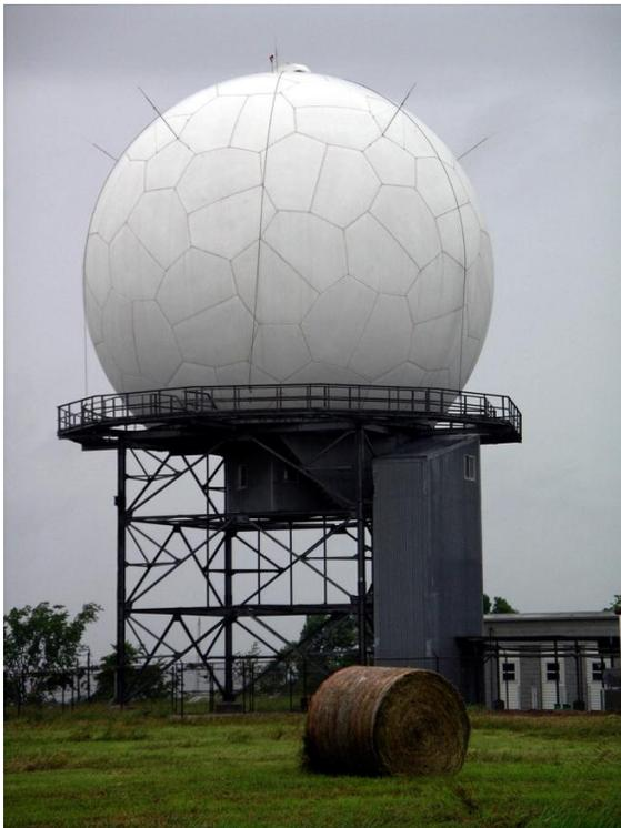
Figure 42. Long-range ARSR (antenna is encapsulated by radome).
