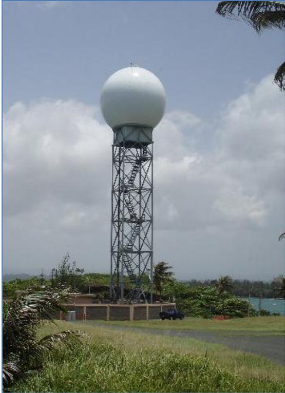
Figure 53. TDWR antenna.
