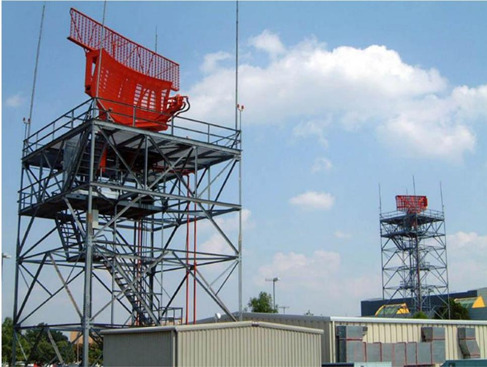
Figure 44. S-band ASR test and research systems.
