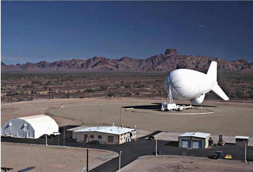
Figure 41. Balloon-mounted Aerostat L-band long-range radar.
