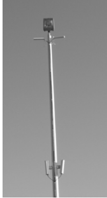
Figure 7 Yagi backbone antennas and sector AP antennas
