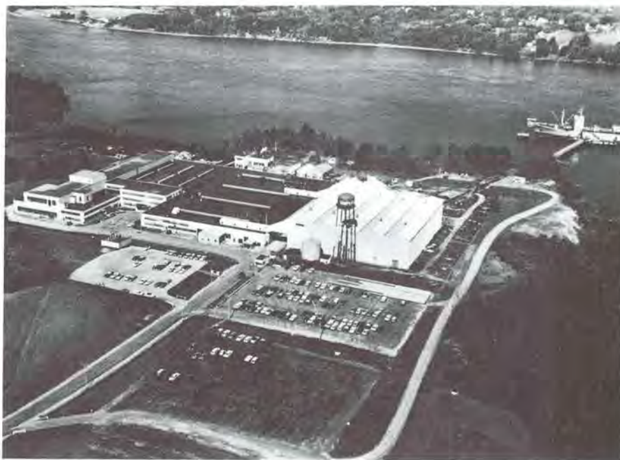
Aerial view of the Simplex Wire and Cable Company plant at Newington, New Hampshire, with cables NEPTUN(3), then the property of United States Underseas Cable Corporation, loading cable for a U.S. military project in Southeast Asia. Since then, Simplex has added an all-weather enclosure to the cable-loading facility so that operations are not impeded by accumulation of ice or snow. Also a new multi-million-dollar addition to the plant was dedicated in 1980 for the development and production of fiber-optic light-guide cable under contract to AT&T.
