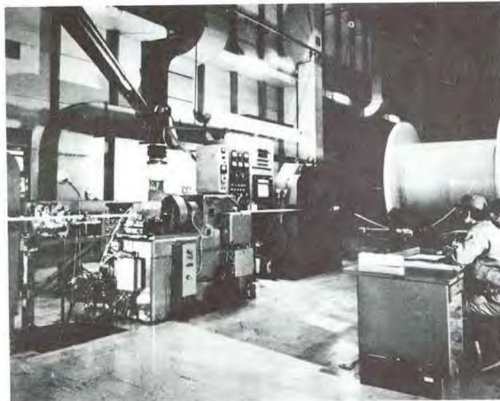
Organized in the late 1960s by a consortium of several large electrical cable makers, Ocean Cable Company Limited's new plant for the production of coaxial submarine telephone cable was established in Yokohama. Under the patronage of Kokusai Denshin Denwa, Japan's international telecommunications carrier, and Nippon Telegraph and Telephone Public Corporation, the domestic carrier, OCC has produced thousands of miles of cable for scores of projects. Seen here is the control center for one of the automated lines for fabrication of the copper and steel center member of the armorless cable.
