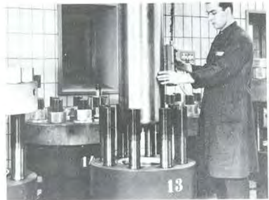
Repeater in Pressure Housing Ready for Helium Leak Test at 750 Atmospheres
