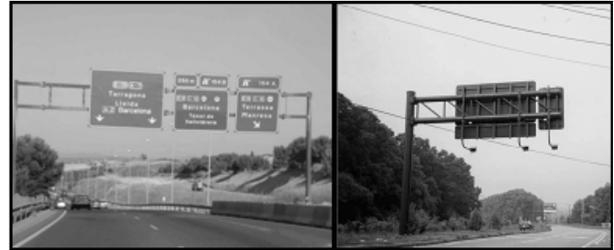
Fig. 4. Examples of sign bridge (on the left) and cantilever sign (on the right)
