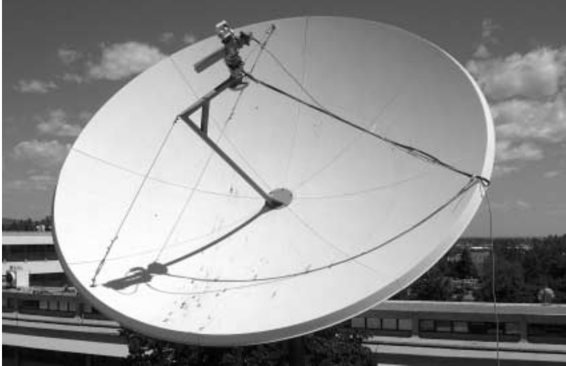
Figure 1. Earth station 3.3-m diameter reflector with RF feed and interference coupler.
